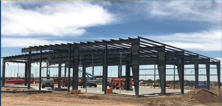
Below: Stage 2 - Steel Framing
